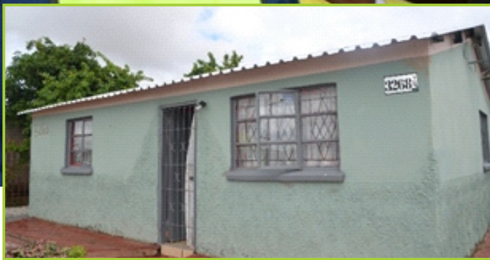
The asbestos roofing of the Thema house in Seshego was replaced with corrugated iron as part of the Department's initiative to ensure an asbestos free Limpopo.
